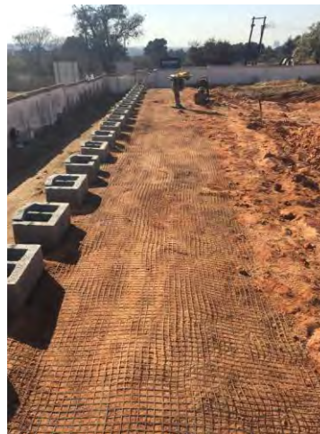
Geogrid reinforced 87 degree wall
